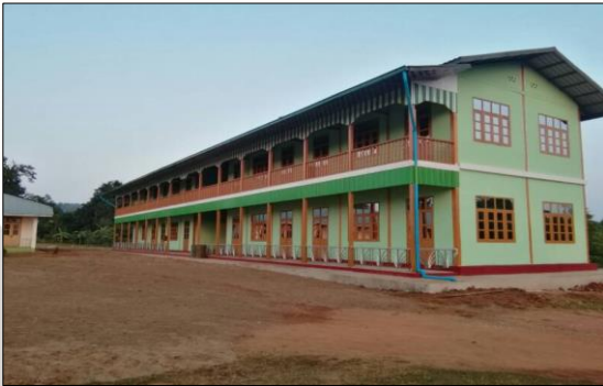
Reconstruction of the School in Lawar Village, Mabain Township, Kachin State
