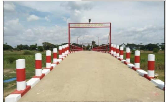
Concrete Bridge in Koe Chin Village, Monywa Township, Sagaing Region
