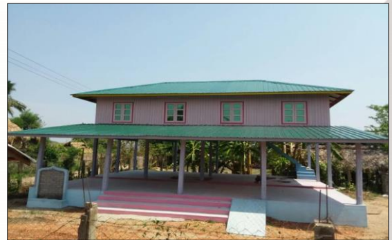
Construction of Rural Community Hall in Ai Taung Village, Kani Township, Sagaing Region
