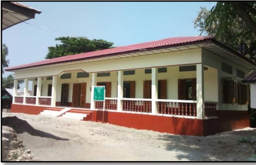
Health Care Centre in Nat Chaung Village, Kalay Township, Sagaing
