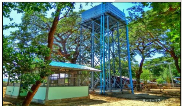
Town Water Supply (Monywa)
