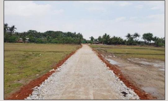
Constructed the Farm Road in Asin Village, Yay Township, Mon State
