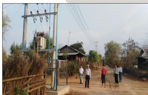
Electrification activities in Sae Village, Ma Hlaing Township, Mandalay Region
