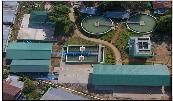
Town Water Supply (Pyay)
