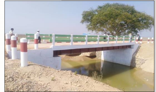
Construction of Farm Bridge in Hton Ai Village, Pha-an Township, Kayin State
