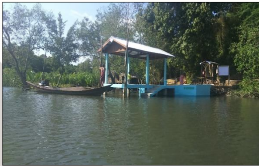
Implementation of Jetty in Ngaputaw Township, Ayeyarwaddy Region
